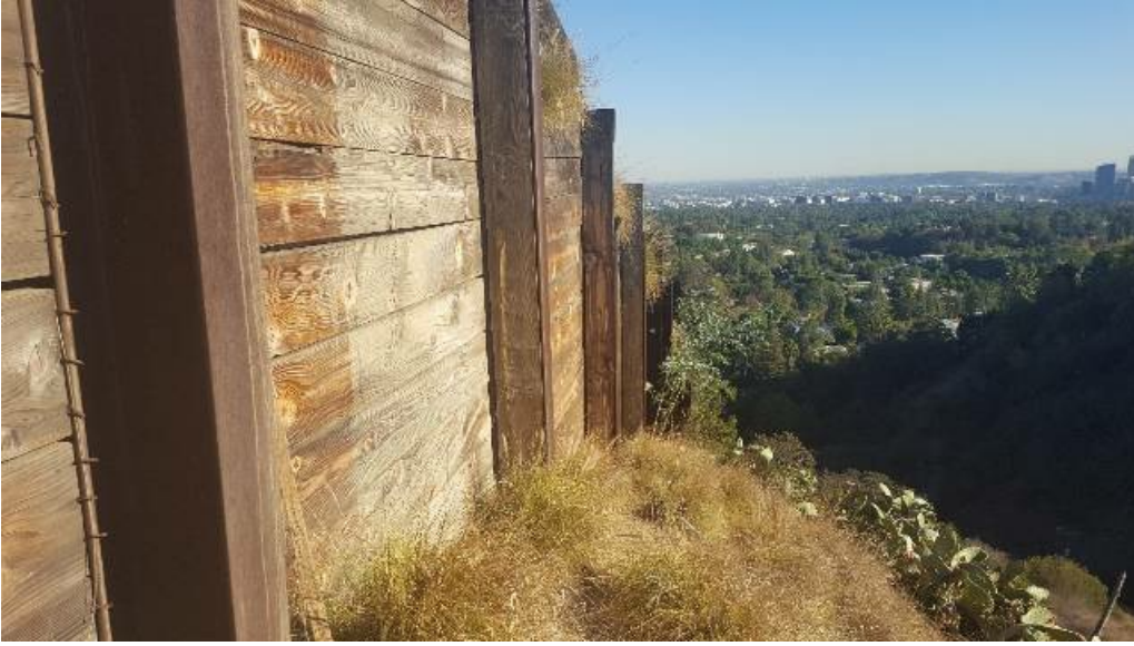
Other: West side shoring
