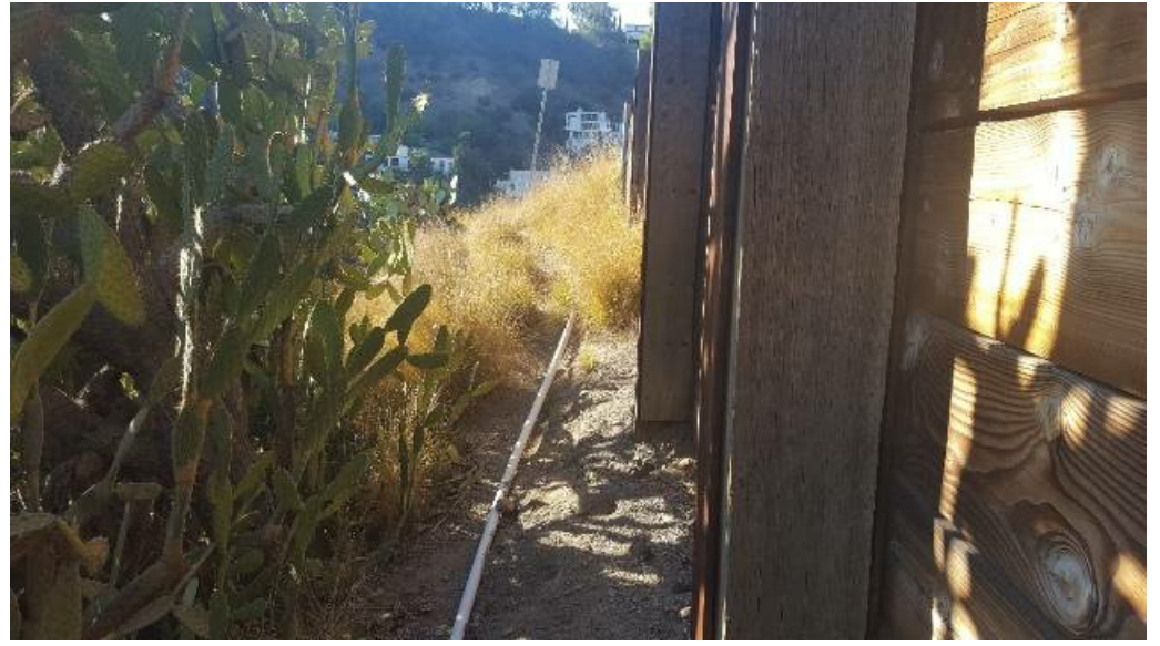
Other: West side shoring retainin
