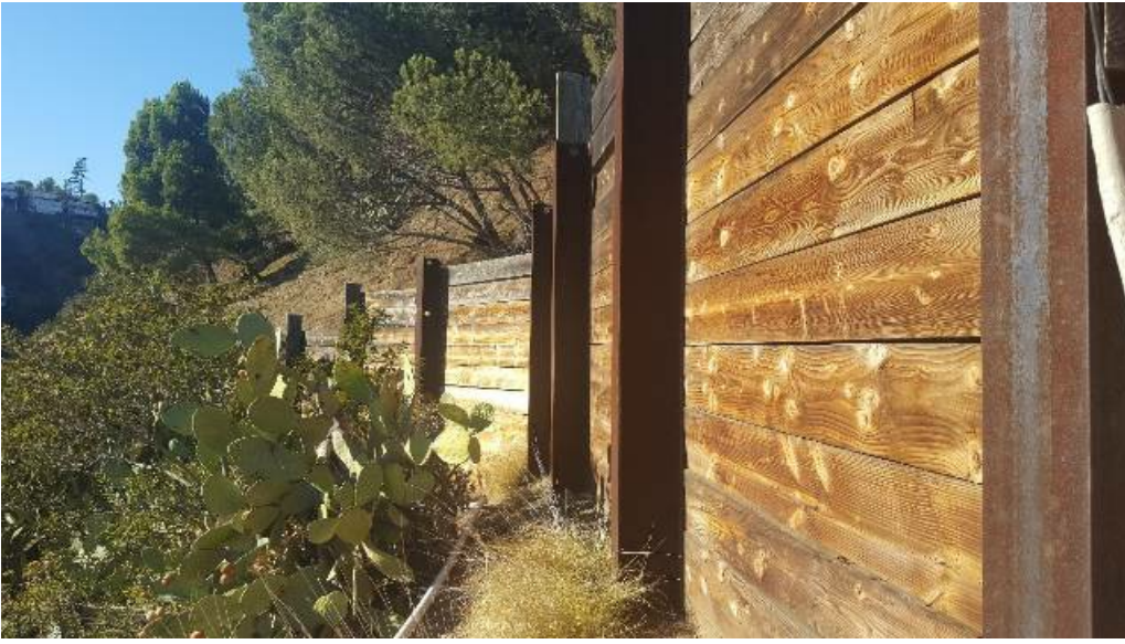
Other: West side shoring retaining
