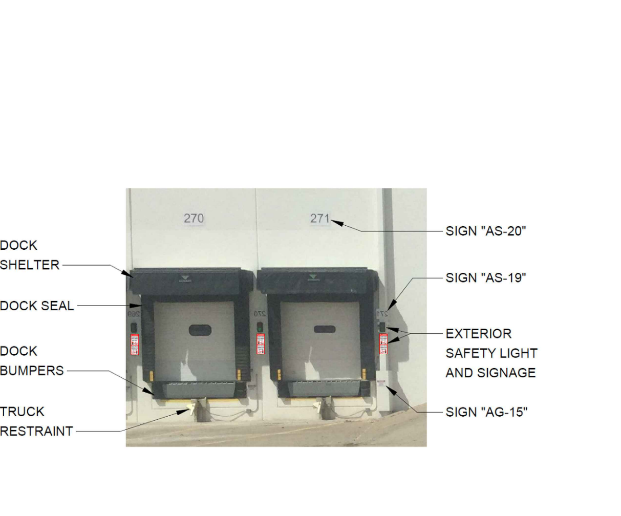
SIGNAGE AT EXTERIOR DOCK SCALE: NTS
